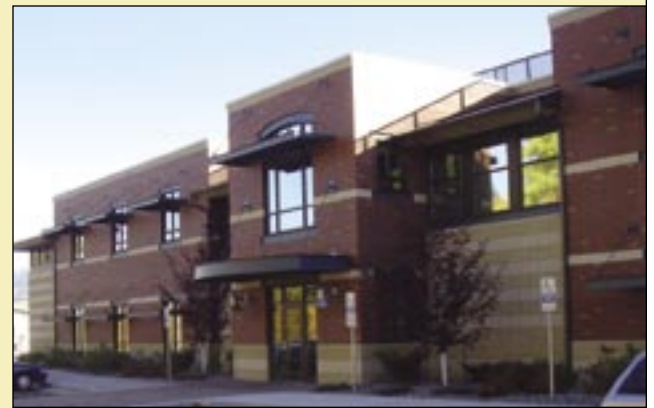
Lattice Materials facility after a recent expansion.
